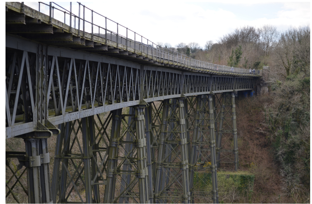
Meldon Viaduct Bridge
